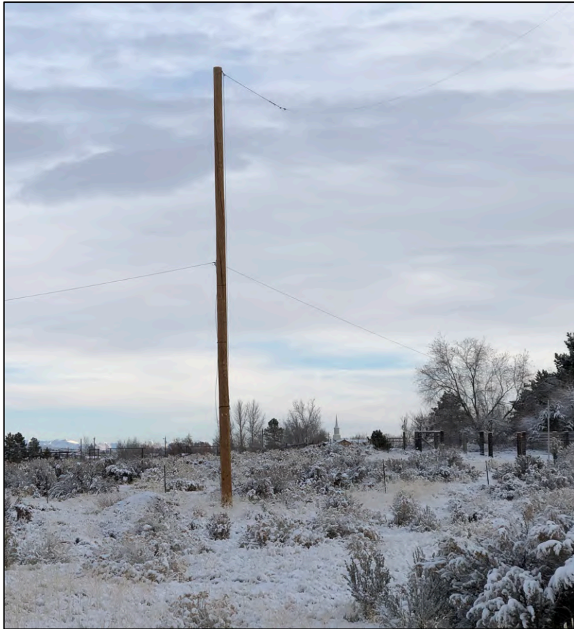
WO7I, N. Nevada: 1.8 to 30MHz OCF Inverted Vee -> 30MHz LPF -> BCB -> LNA (30dB gain, NF 1.8 dB) -> Splitter -> Splitter -> two KiwiSDRs
